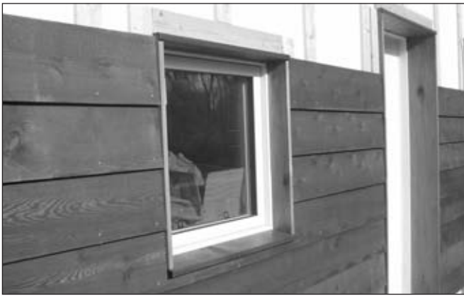
Figure 2. The exterior polystyrene partially laps the window frames. The builder used exterior jamb extensions and wood window sills to trim the edges of the polystyrene and the rainscreen strapping.
