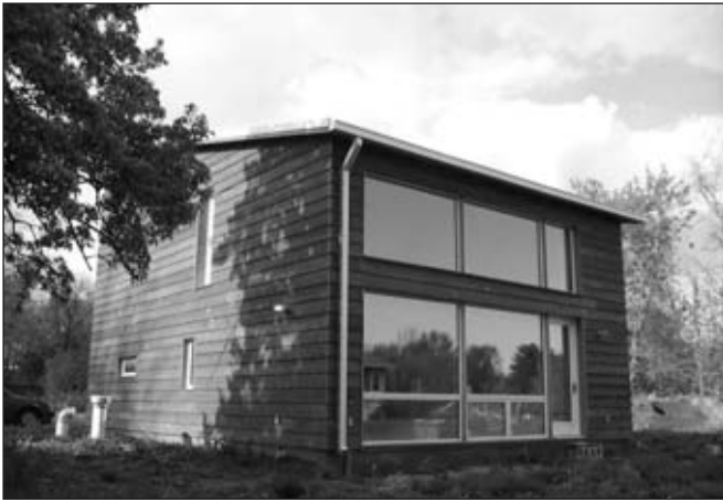
Figure 1. Architect Katrin Klingenberg's superinsulated house in Urbana, Illinois conforms to standards established by the Passivhaus Institut of Darmstadt, Germany. The house's simple, box-like shape minimizes its surface-to-volume ratio. On the west side of the house, the fresh air intake duct and exhaust duct can be seen where they emerge from underground.
