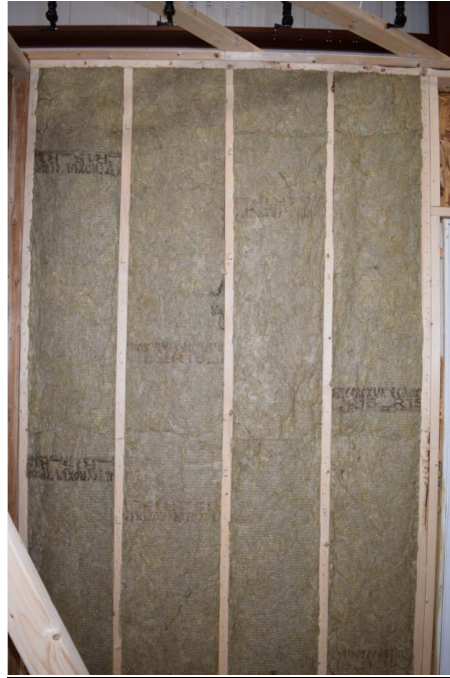
Figure 10. Test Wall with Rock Wool Batt Insulation Installed
