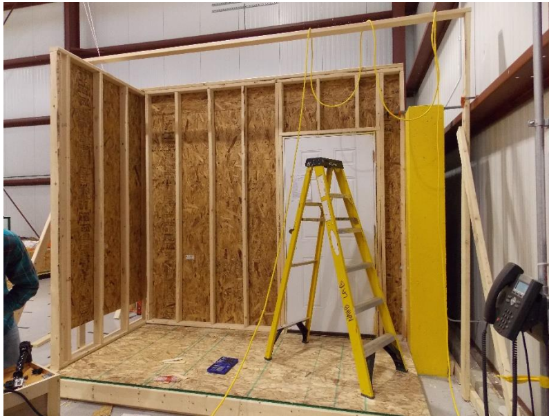
Figure 4. Photo of the Test Wall
