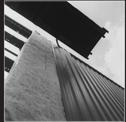
NAIMA 202-96® (Rev. 2000) Certified Fiber Glass Metal Building Insulation is produced in a special manufacturing process to give it the structural integrity it needs to recover thickness after lamination, shipping and installation.
