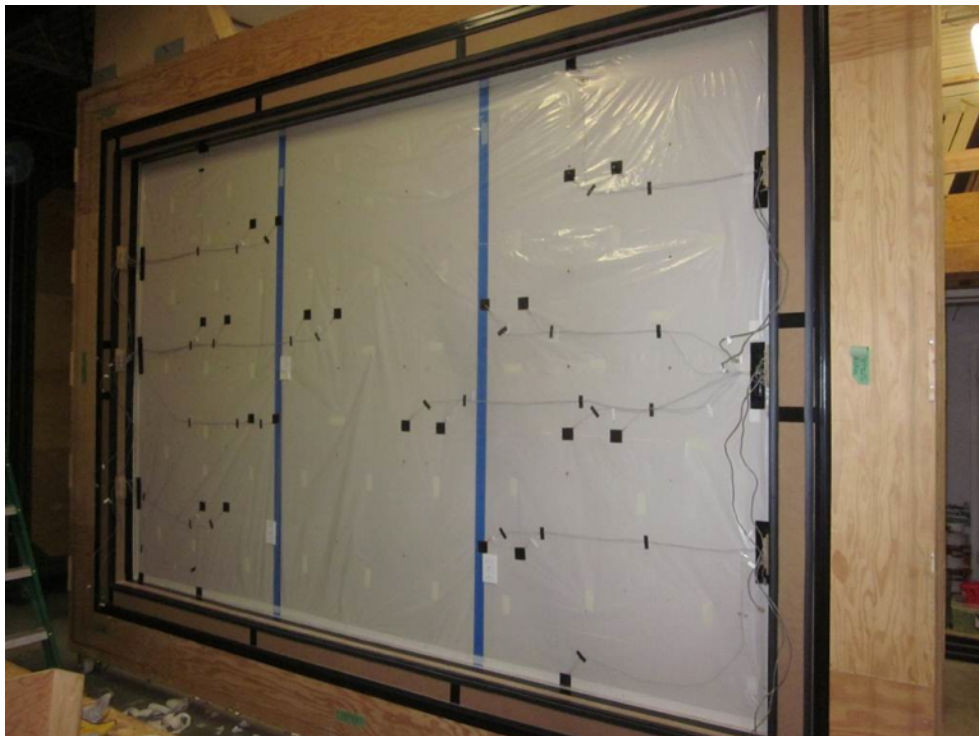
Figure 25 – Meter Box Side, Polyethylene Installed
