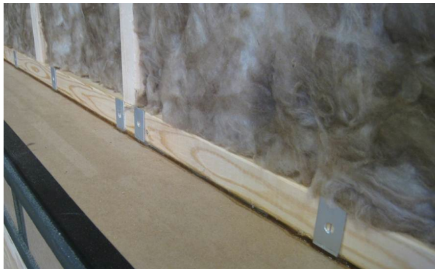
Figure 16 – Drywall Spacers and Fiber Glass Batt Installed
