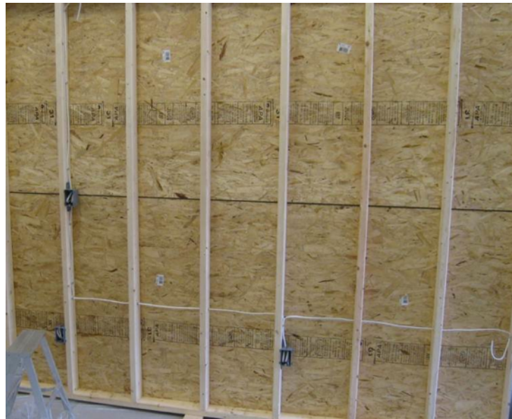
Figure 15 – Electrical Installed and Horizontal Gap Visible
