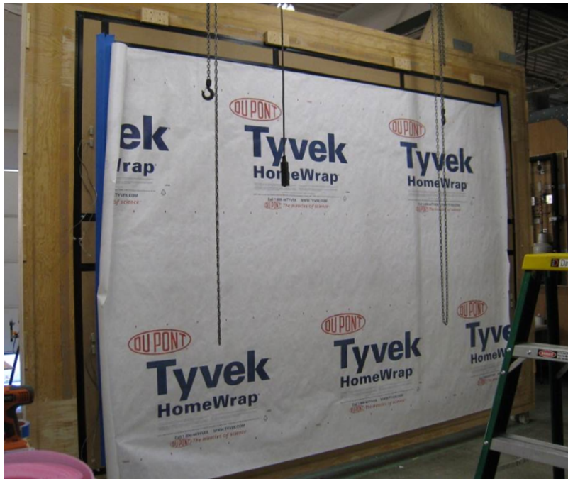
Figure 17 – Tyvek Installed but Untaped
