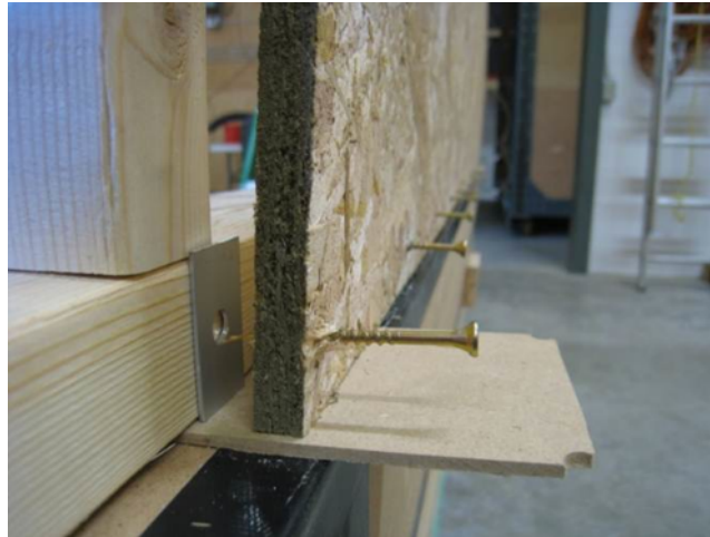
Figure 13 – Spacer Installation
