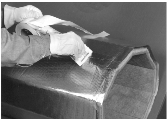
Fig. 3-34C. Taping longitudinal joint of ten sided duct.
