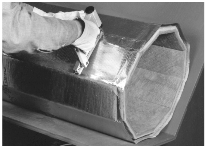
Fig. 3-34B. Stapling longitudinal joint of ten sided duct.
