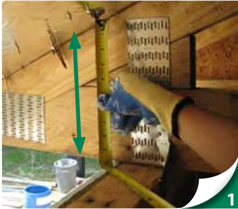
Verify that space between roof deck and top plate will accommodate the appropriate insulation and a minimum 1-inch of required air space.
