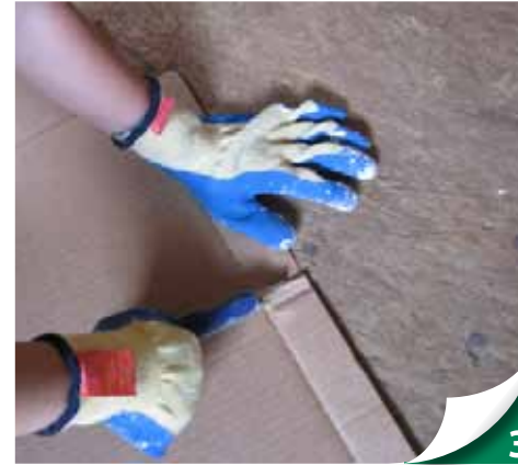
Cut side fin and fold baffle at the measured mark to allow for correct insulation height.
