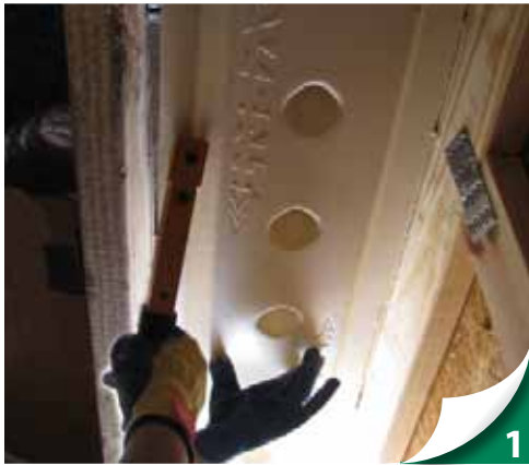
Fasten baffle board to underside of roof deck extending past the outside edge of the top plate and beyond the height of the insulation.
