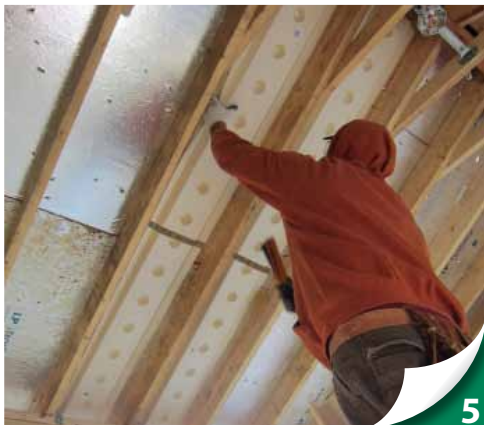
Fasten baffle board to underside of roof deck extending past the outside edge of the top plate and beyond the height of the insulation.
