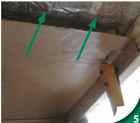
Verify that space between roof deck and top plate will accommodate the appropriate insulation and a minimum 1-inch of required air space.
