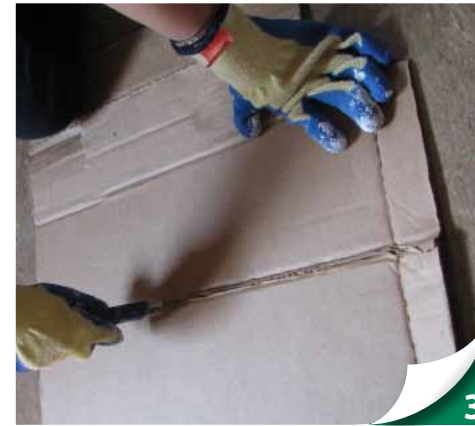
Cut soffit dam material to allow for correct insulation height and any obstructions.
