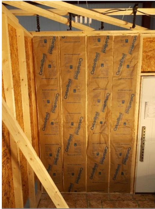
**Figure 10. Test Wall with Kraft Faced Batt Insulation Installed**
