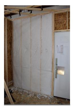
Figure 10. Test Wall with Blown in fiberglass Insulation Installed
