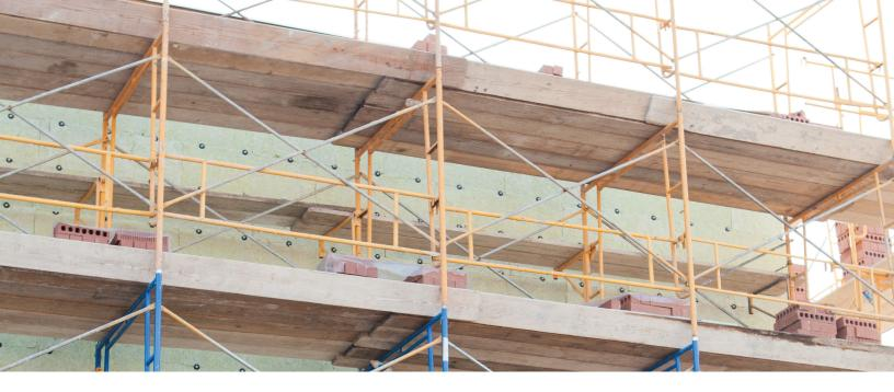
With their very low organic content and their Class A flame spread and smoke-developed ratings when tested per ASTM E84, mineral wool products are ideally suited for use in buildings required to be of noncombustible construction. These products are used as passive fire protection in many buildings and often receive a zero-flame spread and smoke-developed rating—the best possible score—on ASTM E84 tests. The excellent
