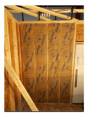
Figure 10. Test Wall with Kraft Faced Batt Insulation Installed
