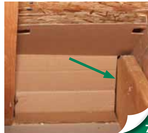
NOTICE: Carefully cut baffle around any framing obstructions to prevent air movement through insulation.
