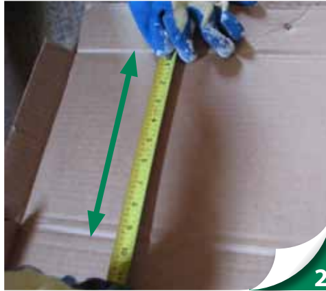
Measure and mark the height on the baffle. Verify the height allows for 1-inch of required air space.
