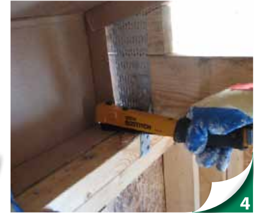
For all eaves with vents, fasten bottom of baffle in place to allow insulation to completely cover the top plate.
