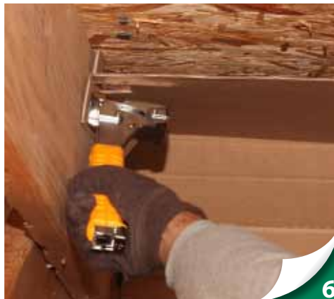
NOTICE: If cathedral ceiling, fasten baffle boards to provide continuous unblocked airflow from soffit vent to ridge vent.
